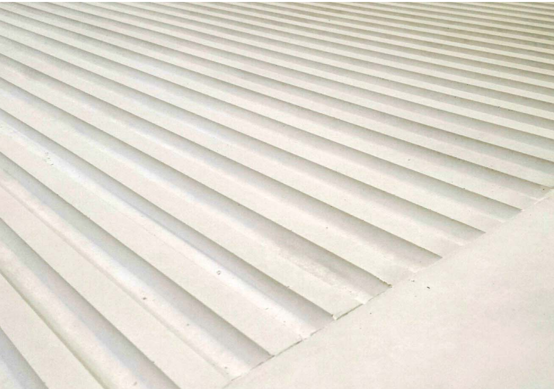
Element with half-stick pattern for project in Copenhagen, Denmark.
