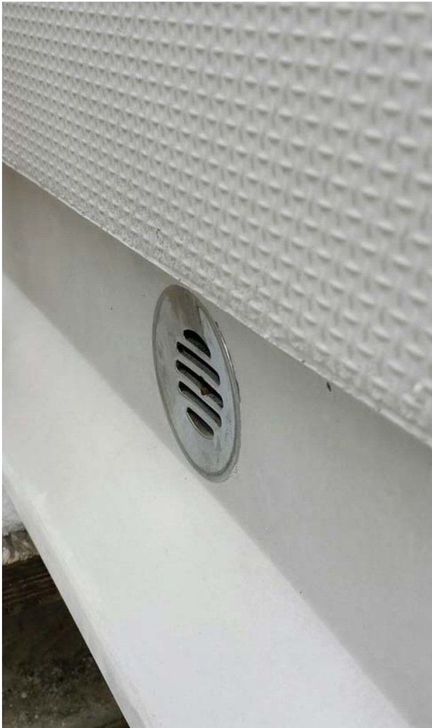
Balcony base with precise mould details of anti-slip surface and water gutter.
