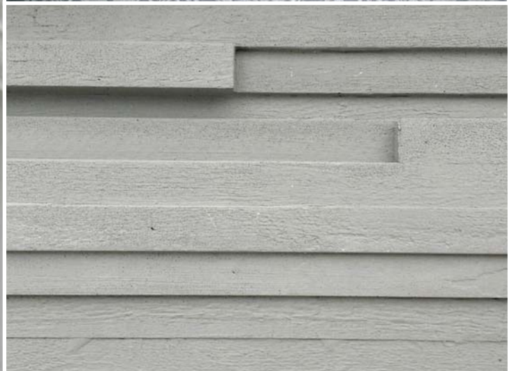
Element for project in Malmö, Sweden with complex mould pattern mimicking wood.
