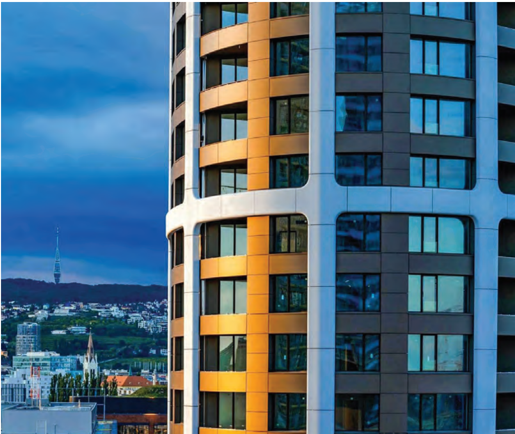
Figure 2: GRC used as exoskeleton at Penta Investment's Sky Park by Zaha Hadid.
