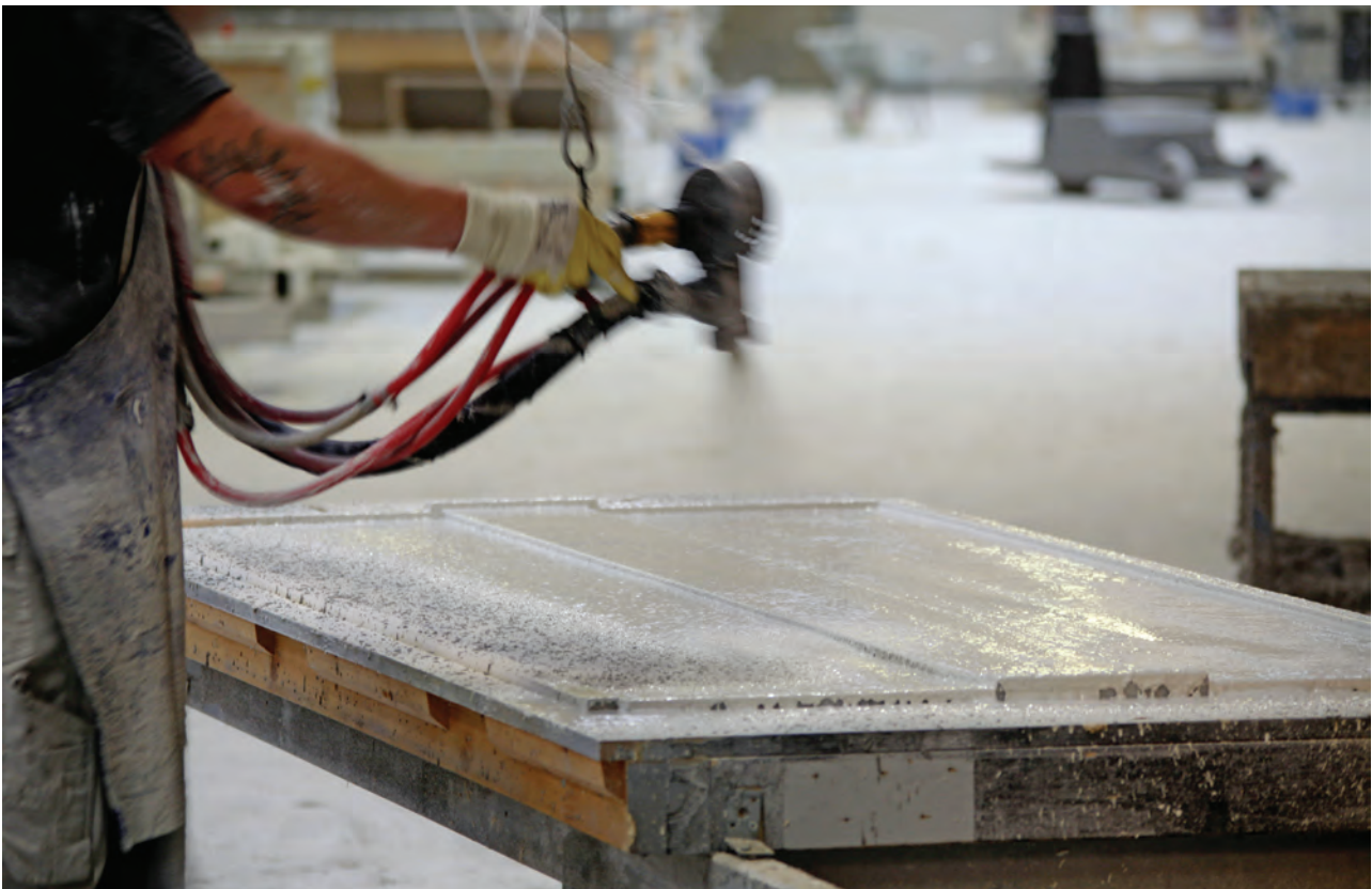
Figure 1: Spray-casting of GRC.
